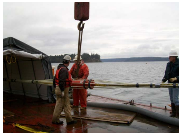
Completed splice being put in water
