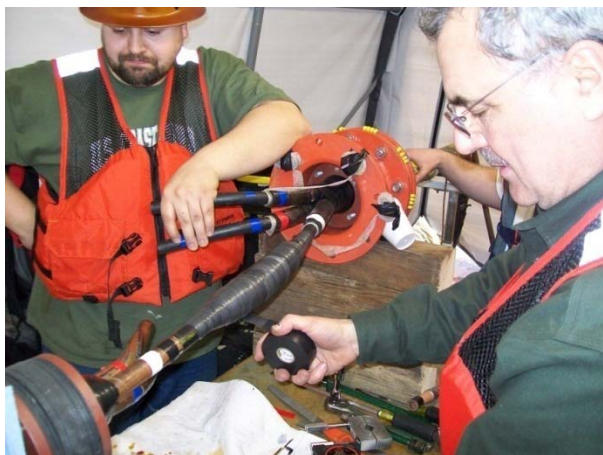
Repair of marine cable by splicing new section
