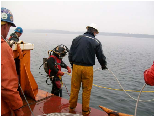
Diver entering the water to retrieve cable
